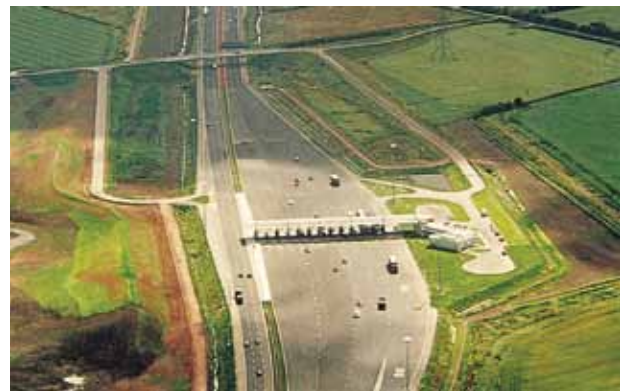
Second Severn Crossing Bridge Toll Plaza, fundamentert med Tensar geonett LTP (UK).
